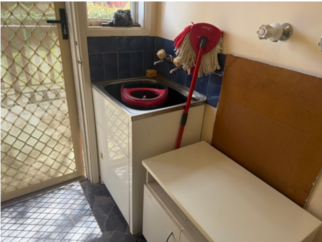
Water pressure tested, is sufficient.
