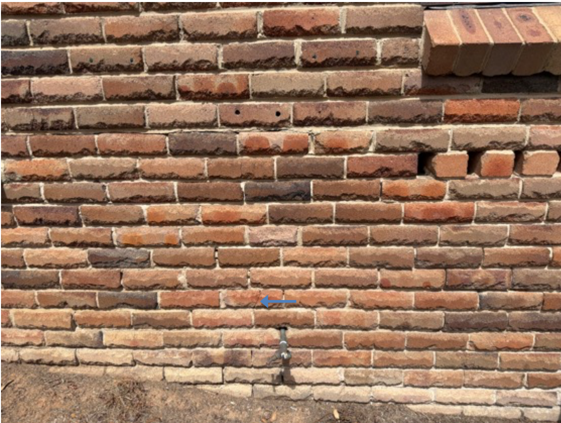
Isolated sections of external brickwork displays category one hairline cracking, rear elevation mid section example above.
