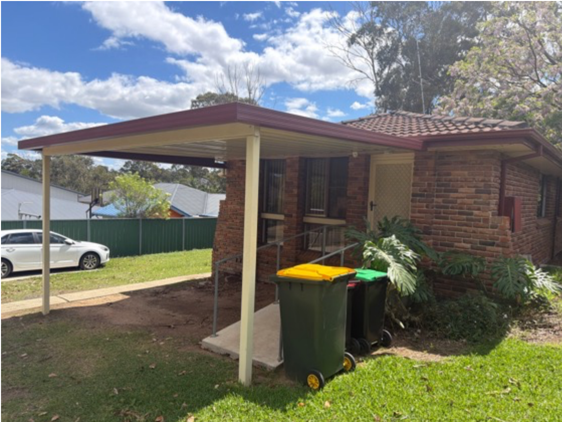
The carport checked is structurally sound.
